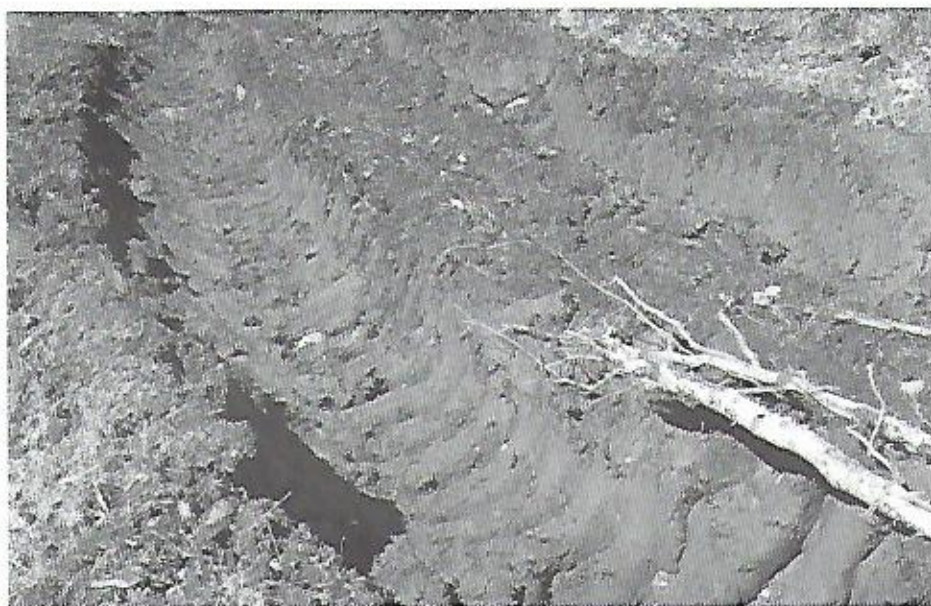
Roads can become heavily rutted during logging, so be sure to have a road restoration clause in your logging contract.
